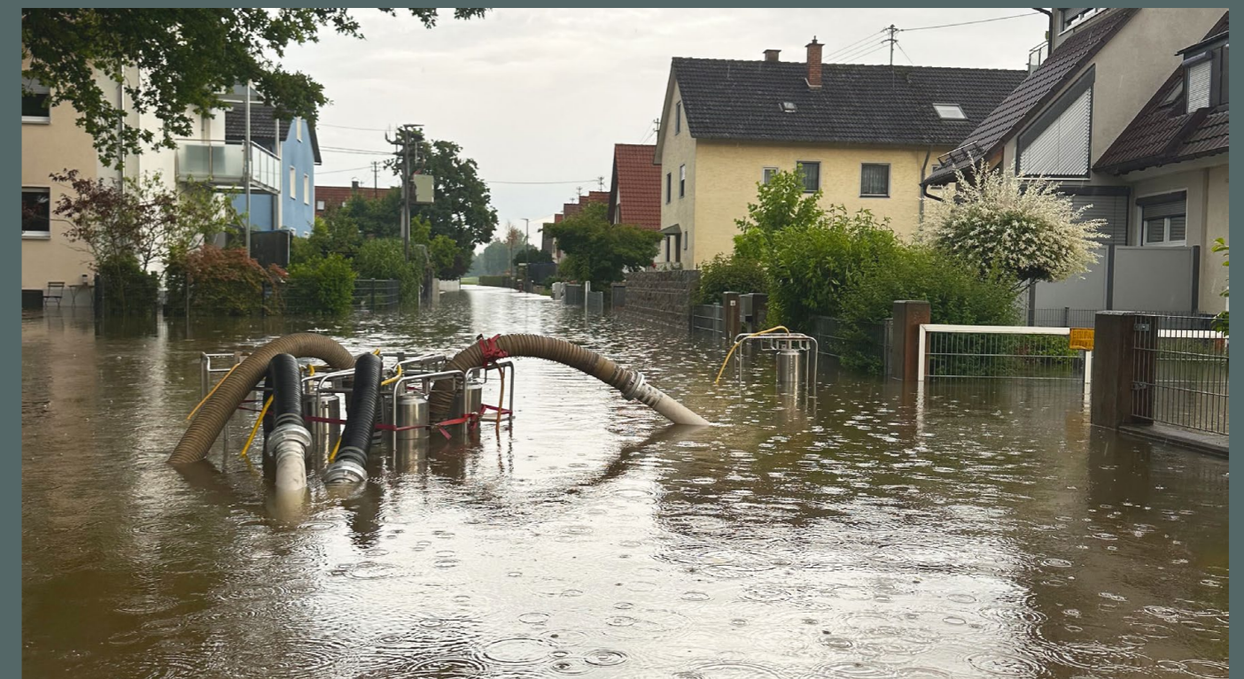
For five days, employees of STAUB & Co. SILBERMANN helped pump off the floodwaters in the Günzburg area.
